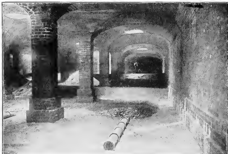
INTERIOR OF A FILTER: DRAIN, GRAVEL AND SAND LAYERS.
